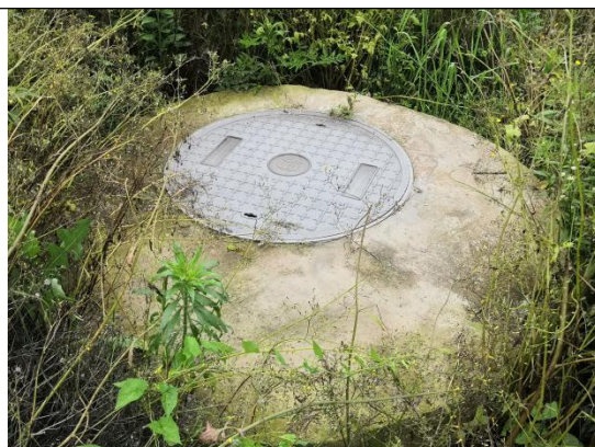
渗滤液监测井
